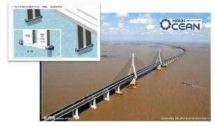
The bridge is 32.5 kilometers long and has 500 piers, each of which can be installed with a 40-kilowatt Drakoo. It can constitute a wave power array of 20 MW. It is estimated that the entire bridge can produce 46 million kwh yearly. If calculated at 75 cents per kw/hour, the total annual power generation is equivalent to 34.5 million yuan.
